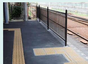
Measures to prevent falls from the platform at Demachiyanagi Station
