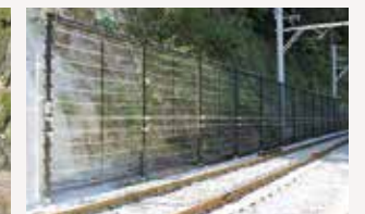
Rockfall protective fences (Eizan Railway)
