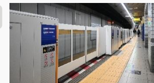
Platform screen doors
